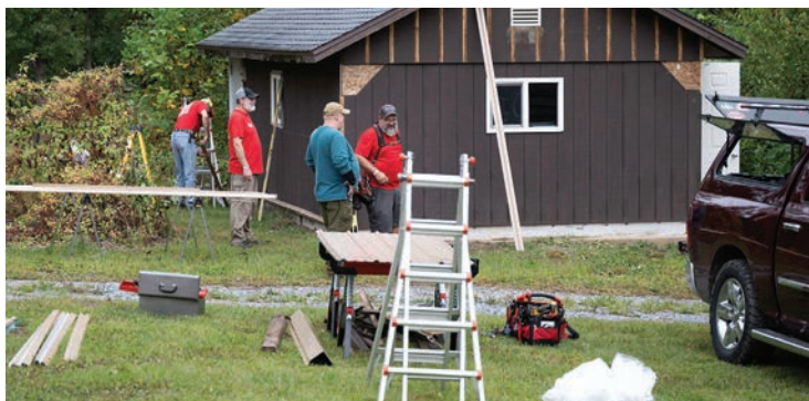
Members working on repairs to the Camp Mack Staff Cabin.
